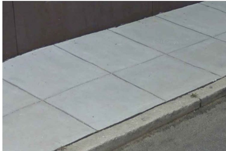
1 DDOT CONCRETE SIDEWALK
